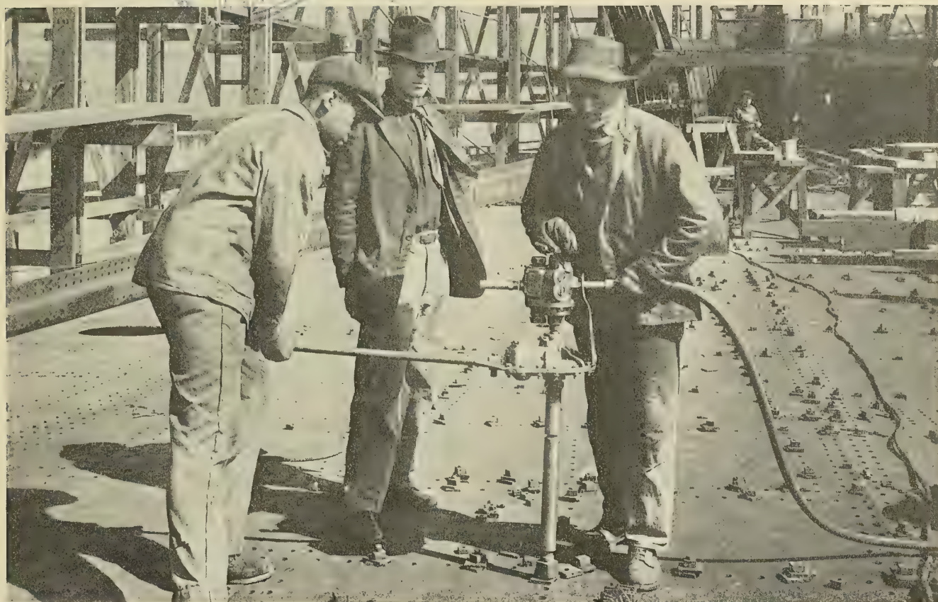
Fig. 1.—“Young” Nut Tightener in Operation
